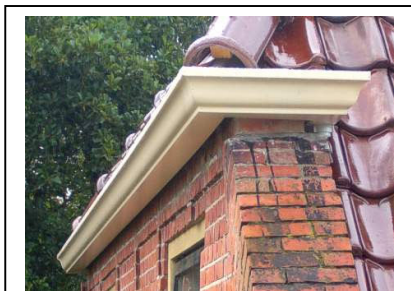
Fig. 1 Aluminium dakgoot
